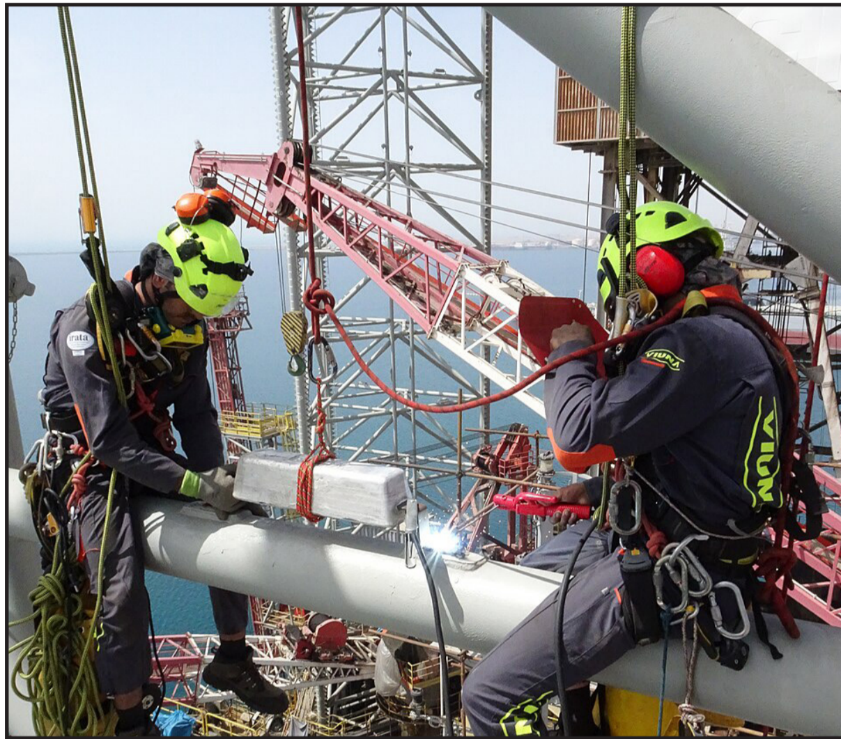
Offshore rig: welders
